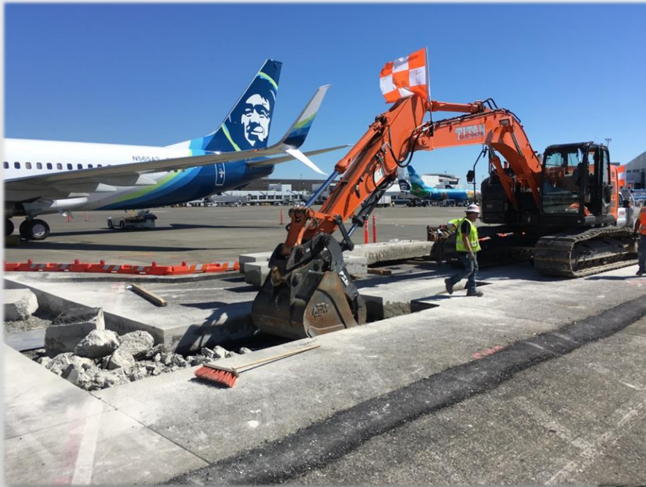
Demolition of ramp
