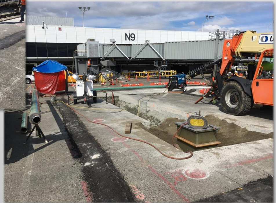
Fuel pit install at N9
